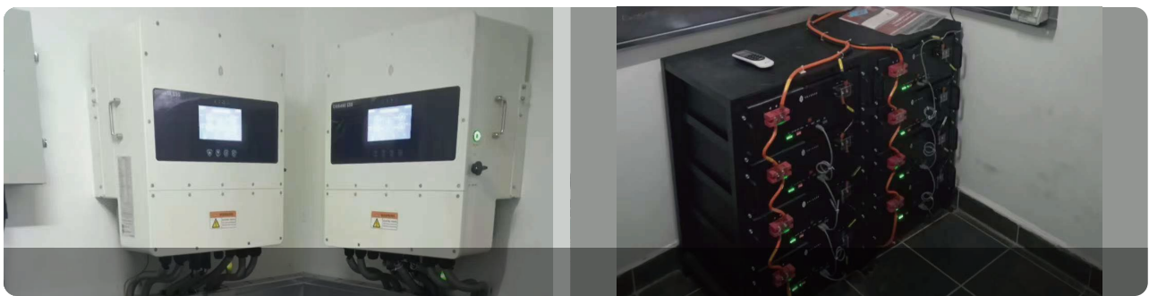
Application: Inverter -- Mars-12G1-LE Battery -- Moon5-R Time: January, 2024 Address: Madagascar Capacity: 12kW*2pcs/5kWh*8pcs
