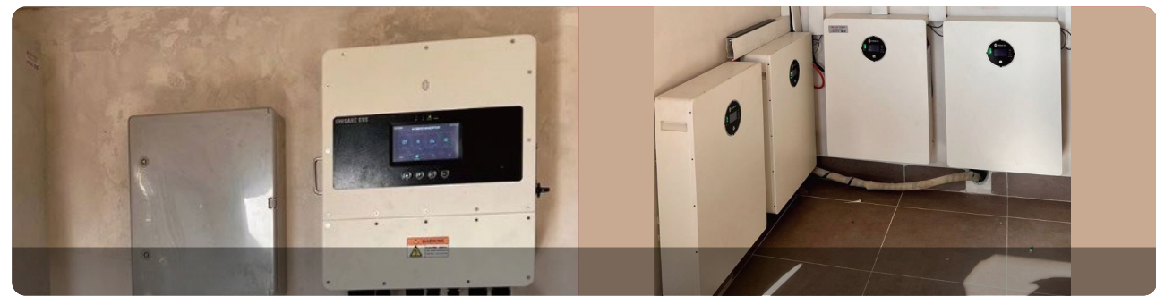
Application: Inverter -- Mars-14G1-LE Battery -- MOONI0-G Time: March,2024 Address: Vietnam Capacity: 14kW/10kWh*4pcs
